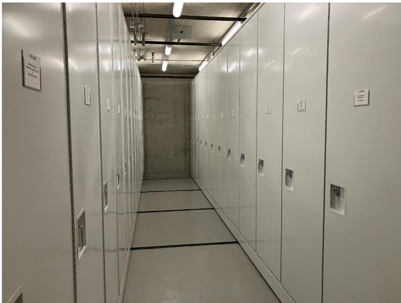
Fig. 1. View of compactors cabinets at CAS.
